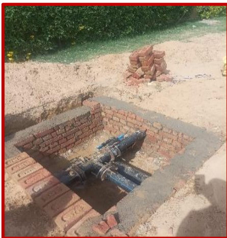
New HDPE pipeline work for PG-1 & PG-2 hostel
